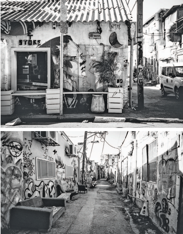
Figure 2. A fragment of the exterior of a building located in the Florentine district of Tel Aviv
