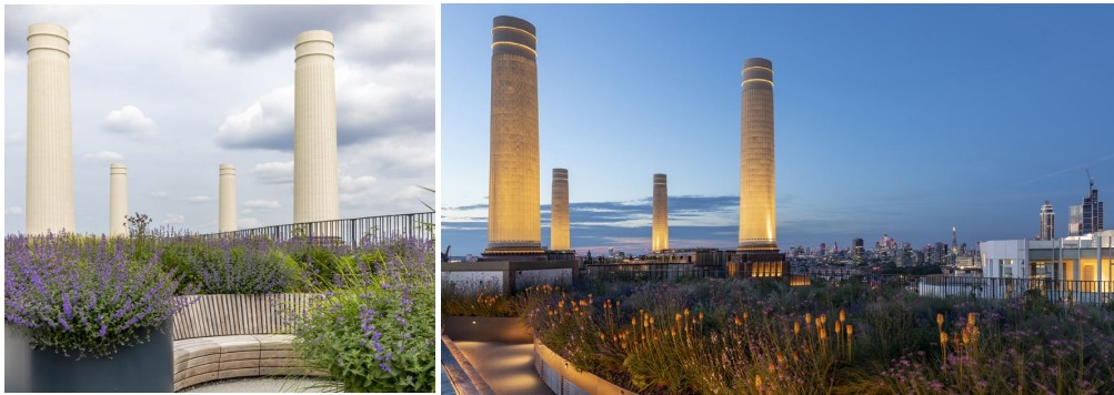
Figure 2. Roof garden at Battersea Power Station
